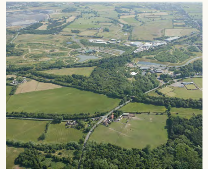
Rawdon Colliery after (Conkers)
