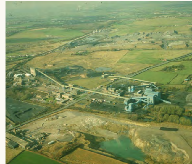
Rawdon Colliery before
